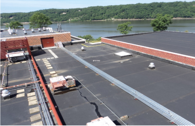
OVERALL VIEW FROM UPPER ROOF AREA...
