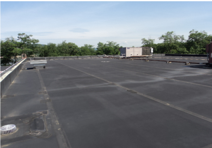
UPPER ROOF AREA...
