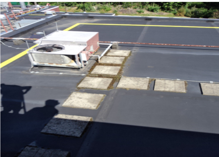
VIEW FROM UPPER ROOF AREA LOOKING DOWN...
