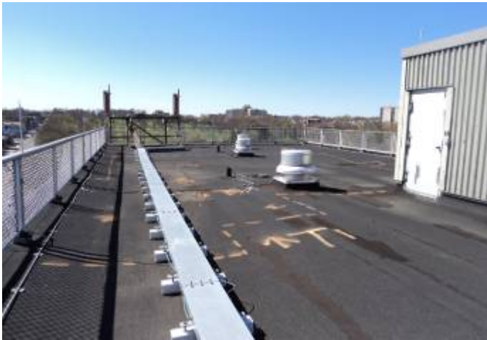
OVERALL VIEW LOOKING WEST...
