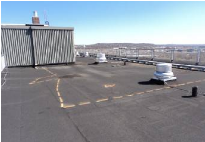
OVERALL VIEW OF 3 LINCOLN LOOKING EAST...
