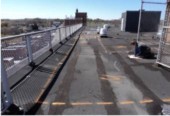
OVERALL VIEW OF 1 LINCOLN LOOKING WEST...
